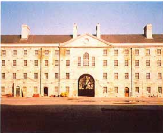
West block during restoration
