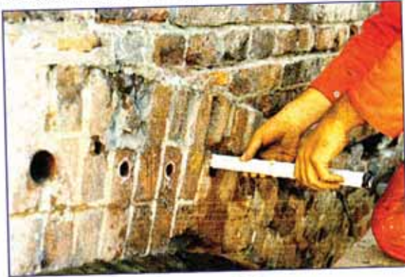
Placing the anchor in the prepared hole
