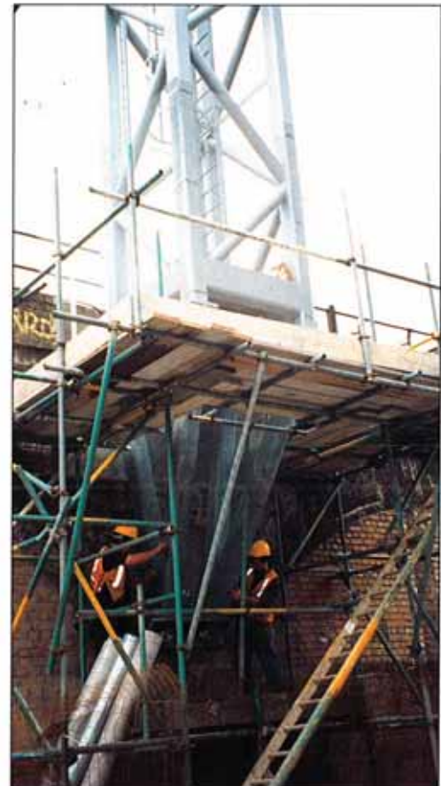
The torquing of the anchors
