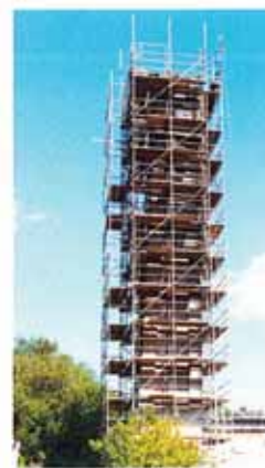
Chimney Restoration In Progress
