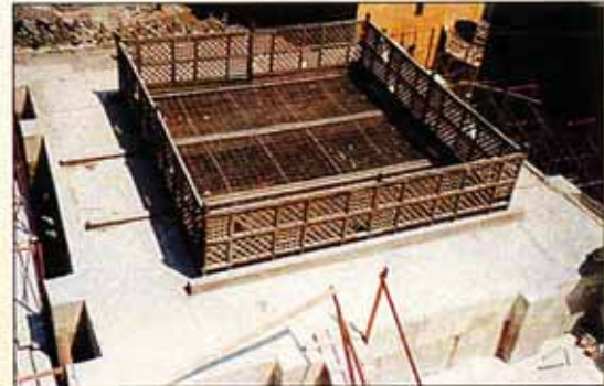
Roof section above central courtyard
