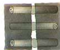
Plan view of stitching anchors
