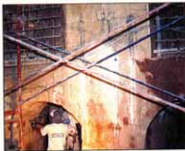
Drilling the vaults
