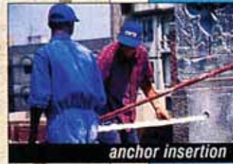
typical consolidation anchor prior to grout injection
