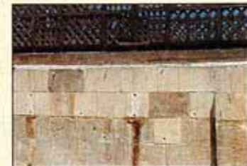
Roof consolidation anchors
