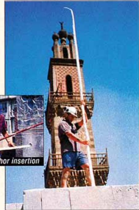
5 metre long vertical anchors at roof level
