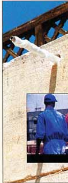
typical consolidation anchor prior to grout injection
