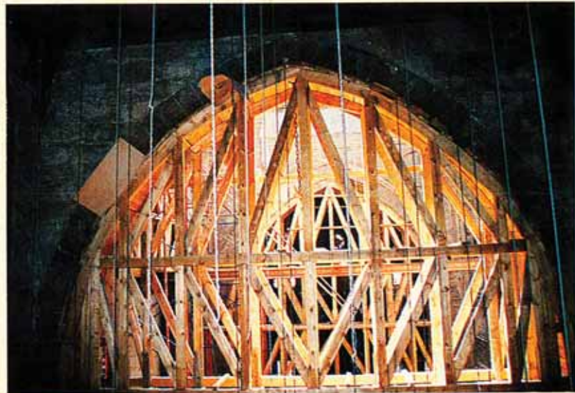
Temporary support of the Dikka arches
