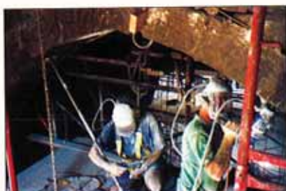
Diamond drilling the arch stones
