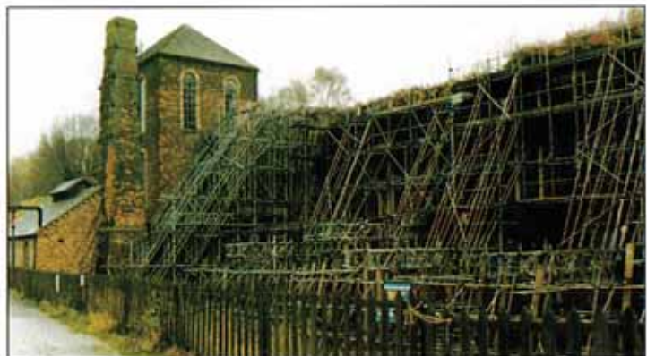
Restoration work in progress
