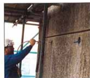
Injecting grout into anchor
