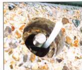
Anchor prior to injection
