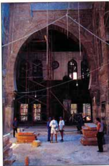
Dikka arch in the main courtyard
